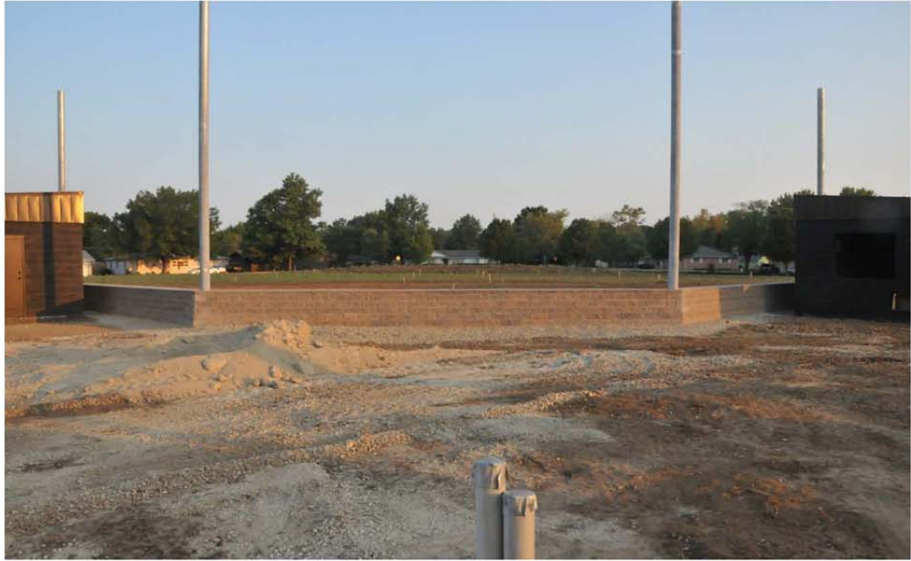
View of backstop wall from bleacher area
