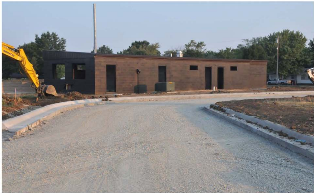
View of curb/drive northwest towards visitor dugout/concessions stand/restrooms
