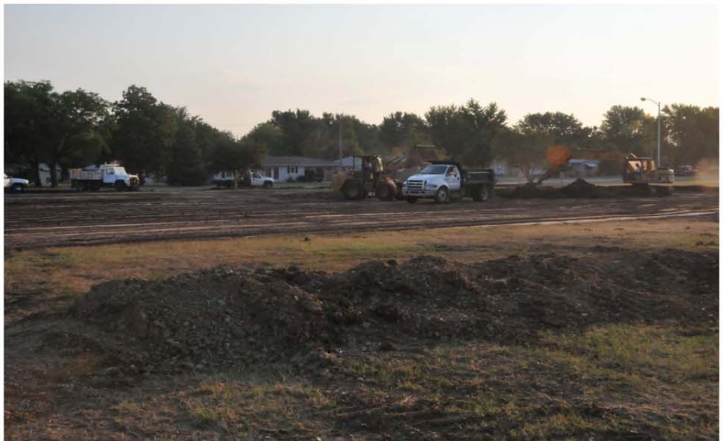
View of north detention basin in progress
