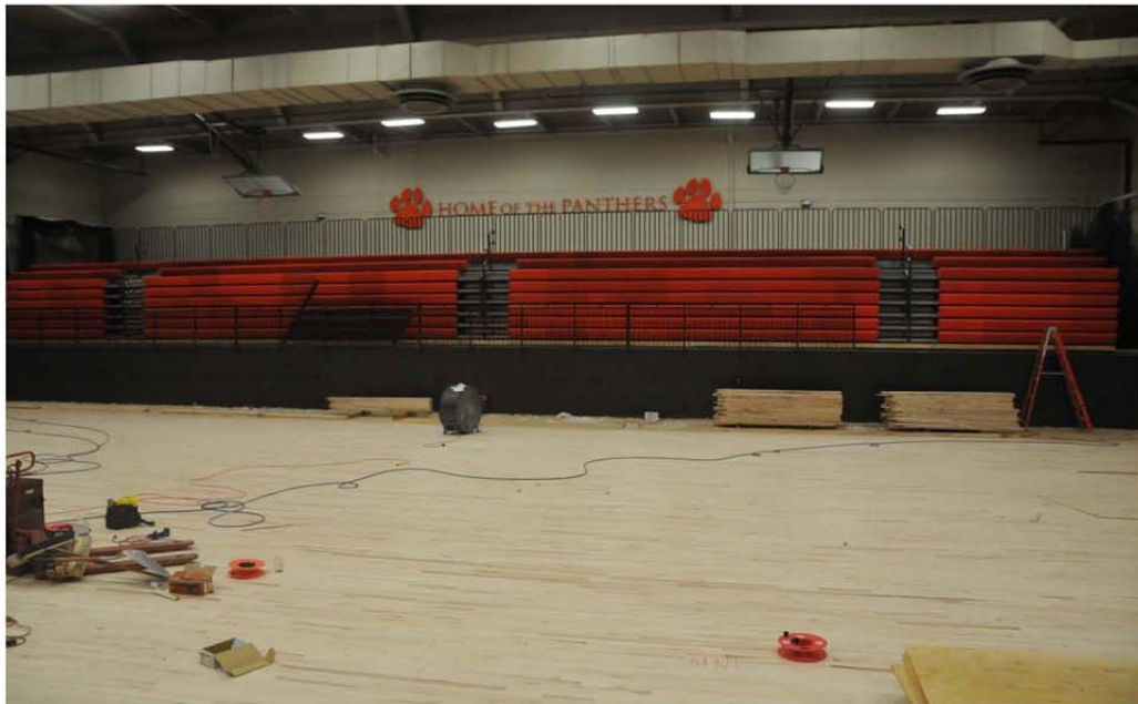
View of mezzanine bleachers and new railings
