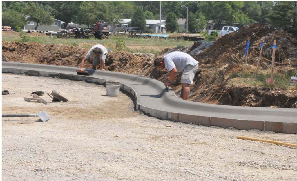
View of R&S Construction workers forming and cleaning curbing
