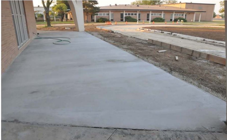
View of replaced Chapman Library porch
