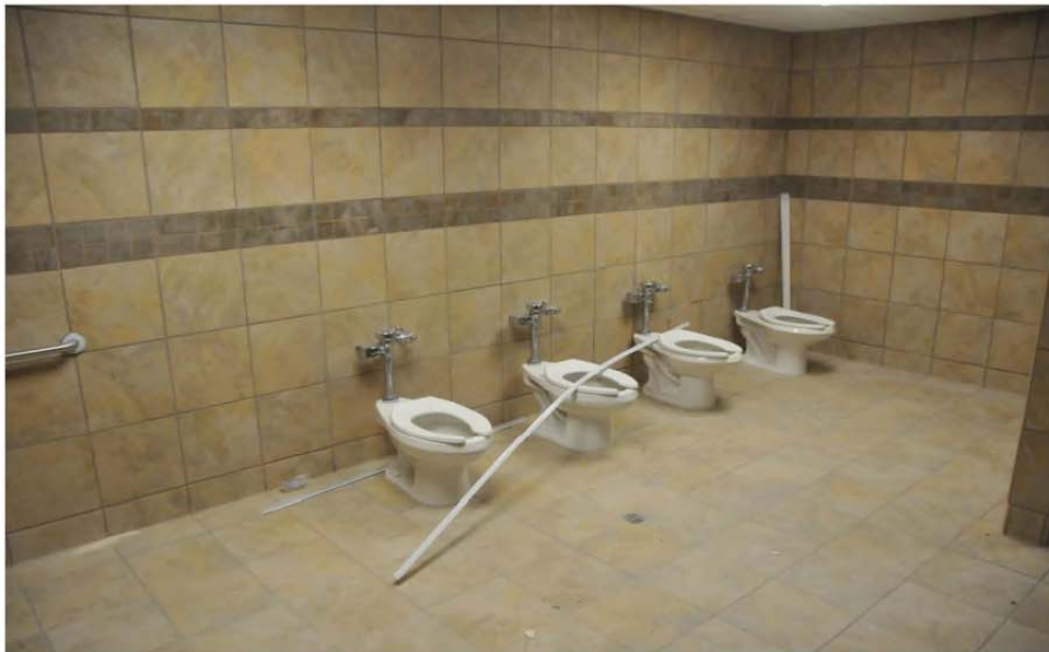
View of ceramic tiles in student union women's restroom
