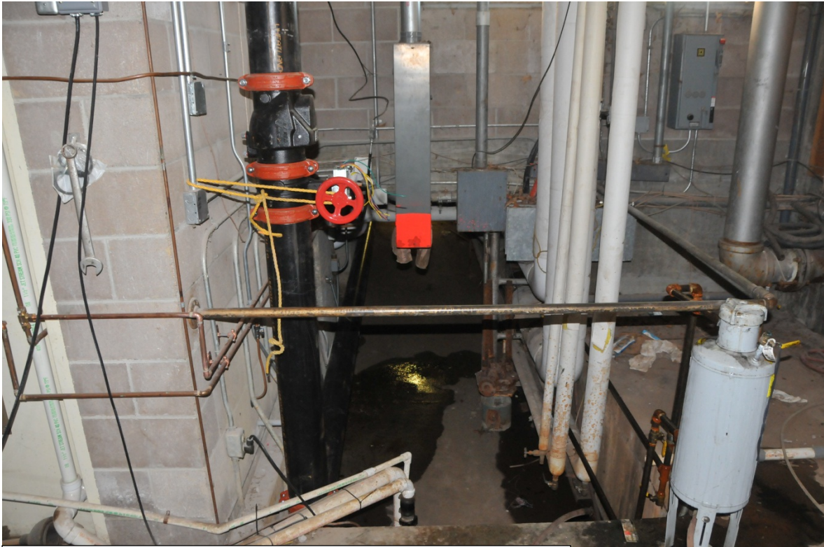
View of sprinkler shutoff at mouth of underground tunnel
