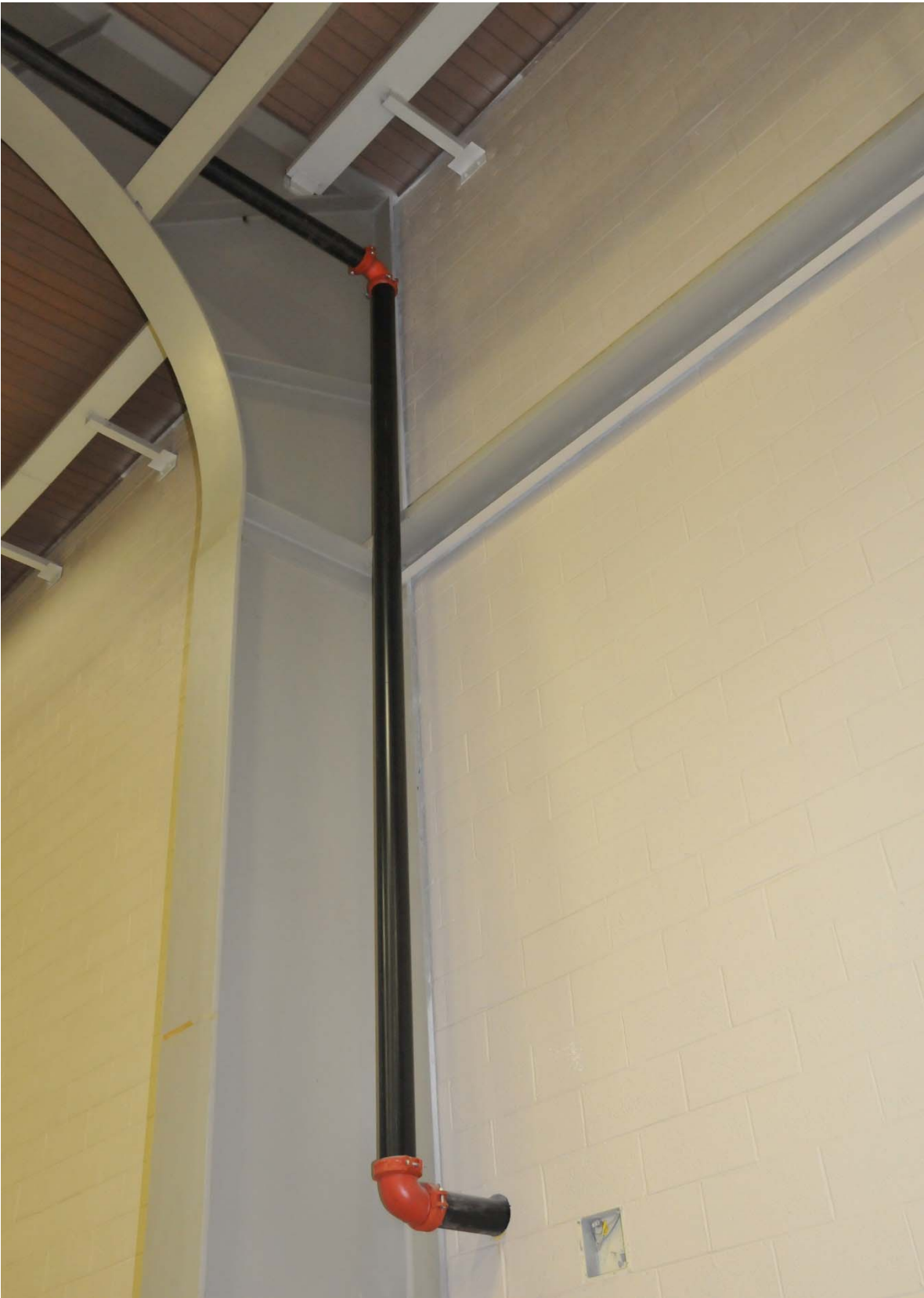
View of sprinkler main in gym
