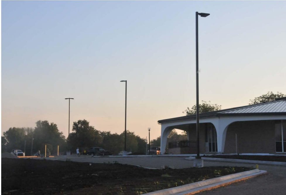
View of drive and new lights
