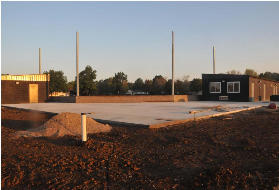
View of dugouts from driveway
