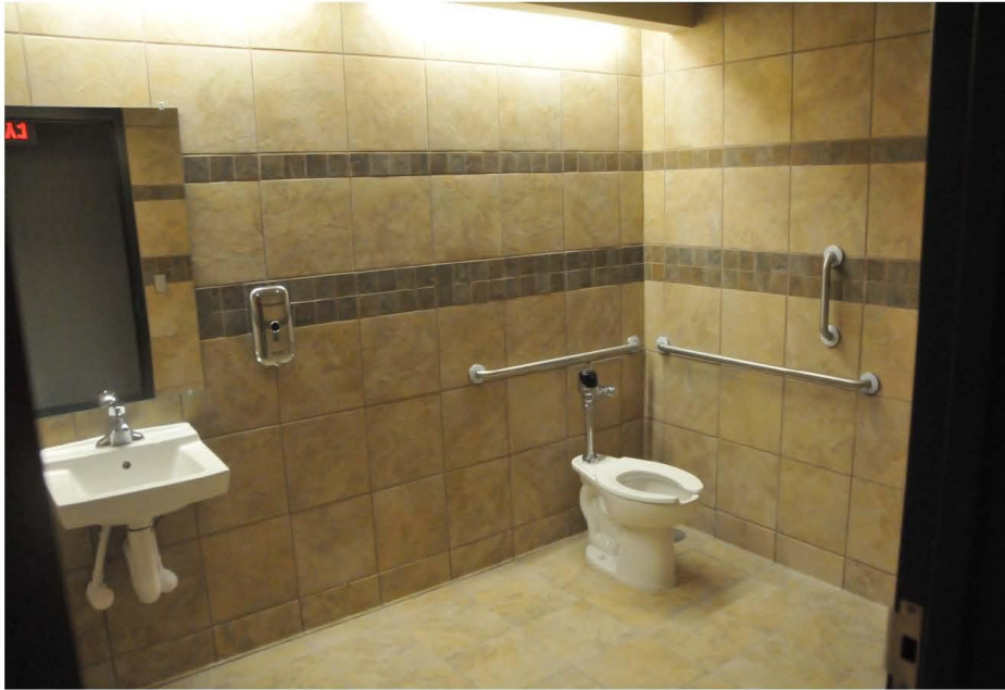
View of men's locker room restroom
